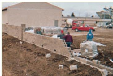
The freestanding StoneHedge® XL wall was also designed to resist up to an 80 mph wind load. A 4" x 4" Anchor Bar on each block effectively creates a mechanical connection with a high shear resistance, making the wall a secure barrier for the plant. A concrete footing for the base course offers stability for the wall and helps prevent settlement. This footing also increased the efficiency of installation.
